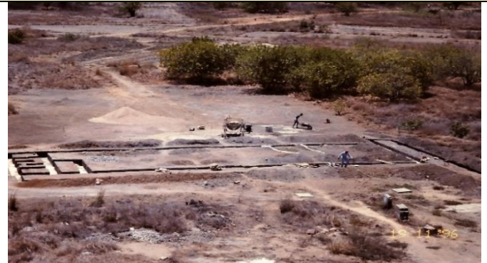
The Foundations for the 1 st Ward
